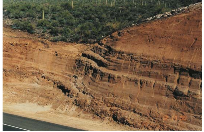
Figure 6. Drainage layback, in this case with ledding and machine scar removal using a plate bucket, followed by staining
