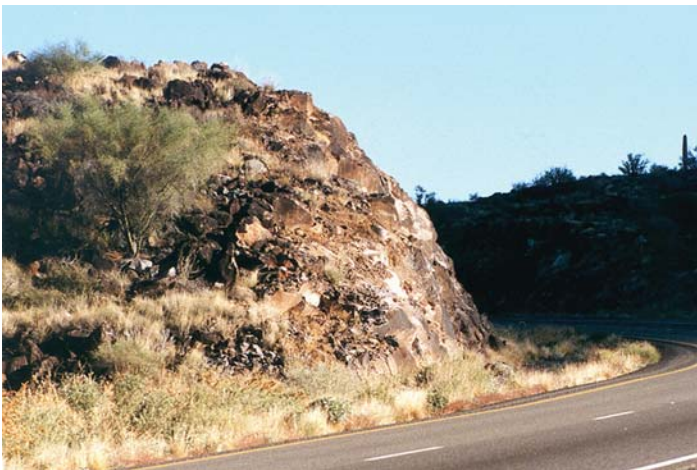
Figure 5. Accentuated rounding. Note how the rounding extends behind the nominal catch point, giving a smoother, natural transition.
