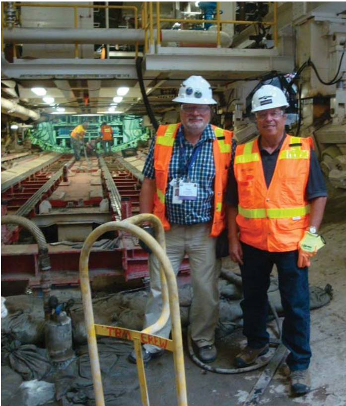
Inside Seattle's Bertha - the worlds largest TBM
