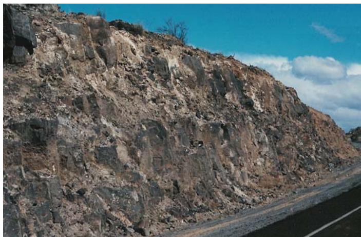
Figure 3. Slope in basalt that was blasted using a cushion technique that reduced back slope disturbance but left a few drill hole traces. However these traces are not apparent from the vehicle occupants' perspective.
