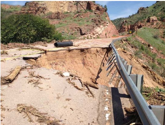
Damage to old U.S. Highway 24 west of Manitou Springs caused by flash flooding from a storm on August 9, 2013, falling on slopes burned by the 2012 Waldo Canyon Fire
