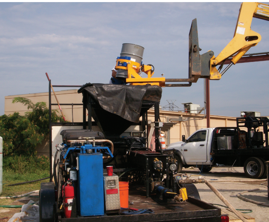
The \text{KMnO}_4 solids are delivered to the fractured well cavity via a steel drum.
