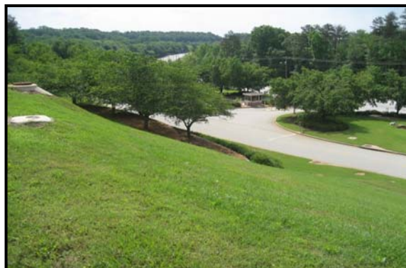
Source Area and Access Road
