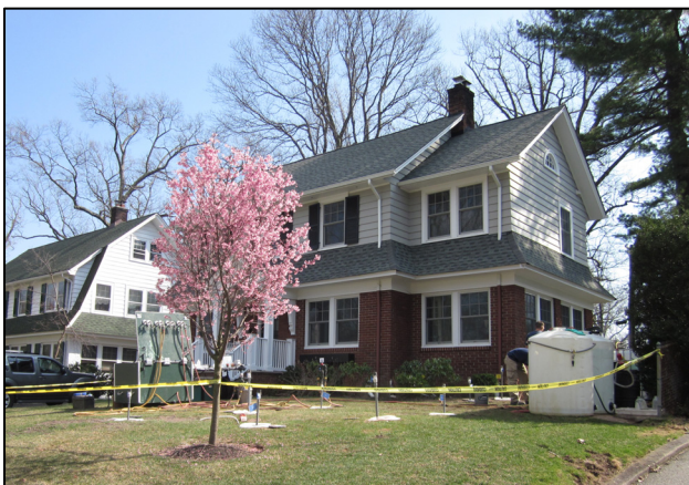
Residential Property during Injection
