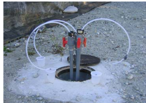
Stick-up injection wells.
