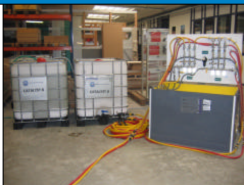
INJECTION SYSTEM INSIDE ACTIVE FACILITY
